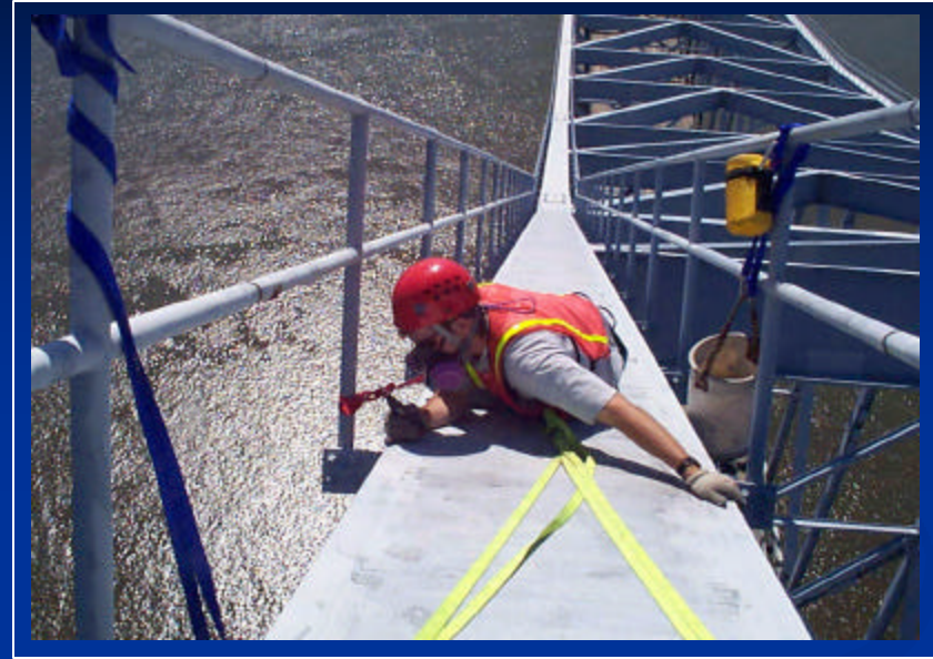
Sensor Installation at Tower
