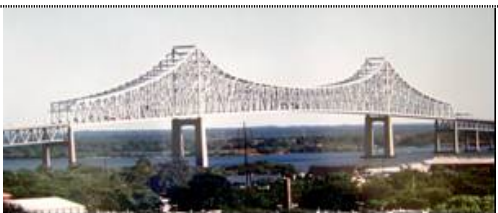
a) Comprehensive Structural Health Monitoring of Commodore Barry Bridge
