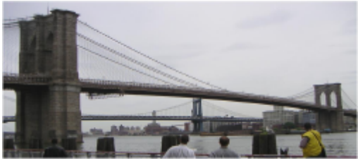
c) Monitoring and Evaluating of Brooklyn Bridge Towers and Deck
